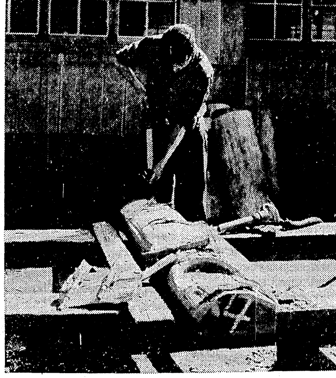
As part of the broadened program in the civilian conservation corps, emphasis is being placed on instruction and training of the young men. Here one is shown at work with an air-driven chisel in the Lower Cispus camp roughing out a rustic table.
